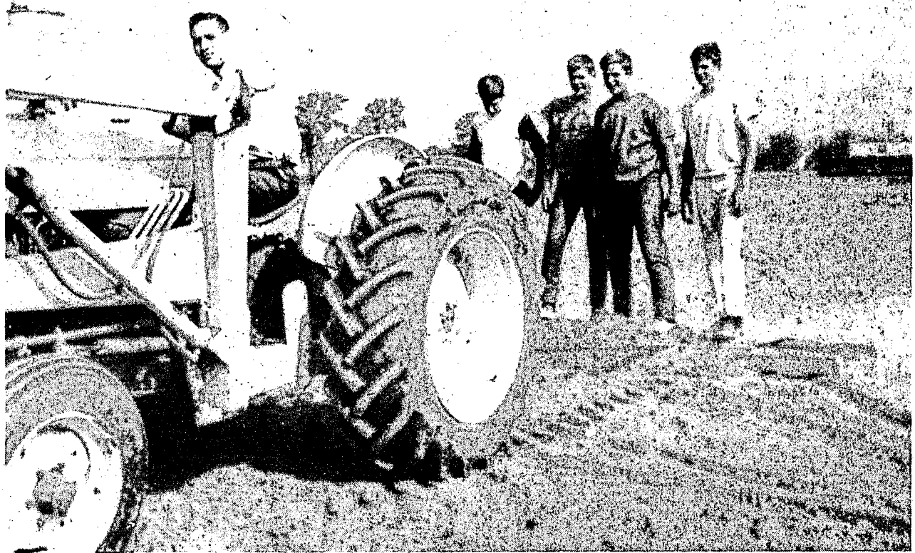
Next spring when the grass is green on this new Senior High school baseball diamond, this crew can say they remember the day they stood on the drag and helped . . . in their own heavy way.
