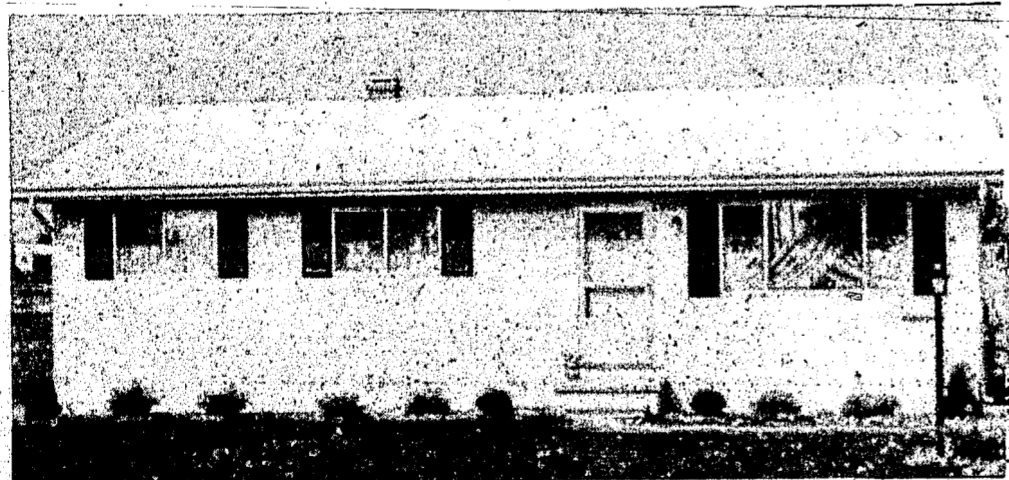
Completed Ranch Home built by Auburn Builders at 6525 Walters Road, Clarkston, Mich.
