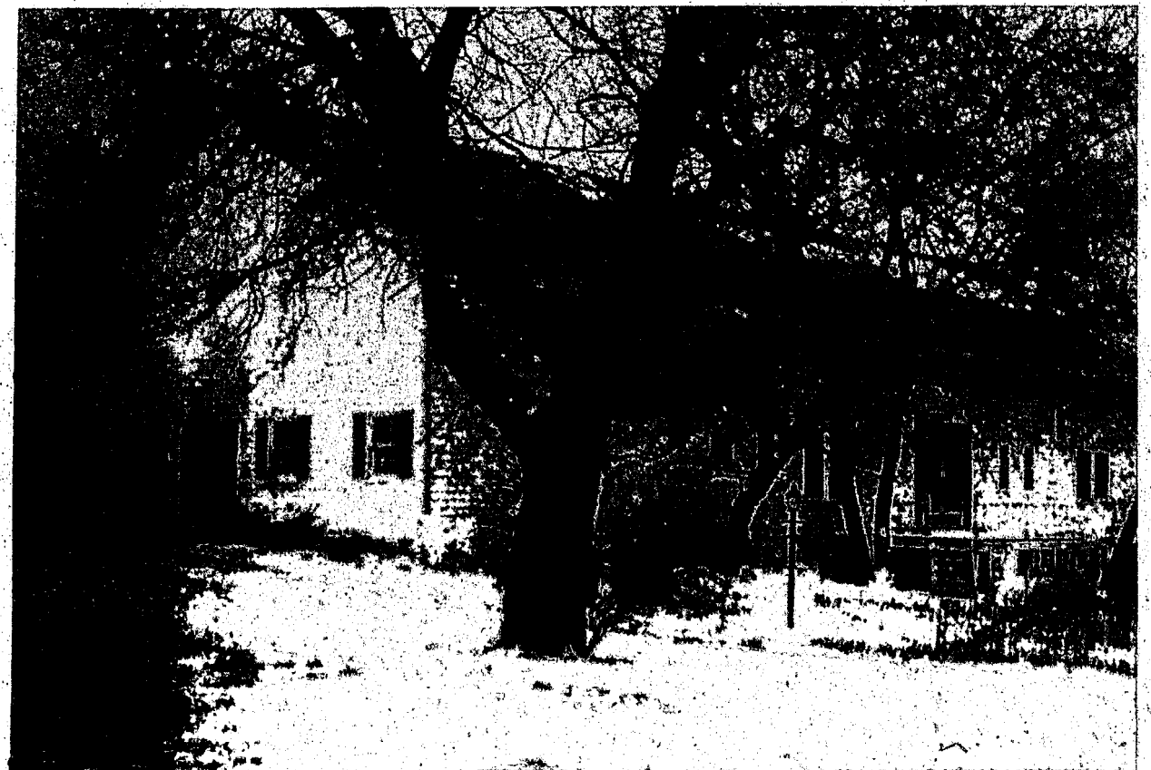
Exterior of the Arthur Rose home, used at one time as a barn.
