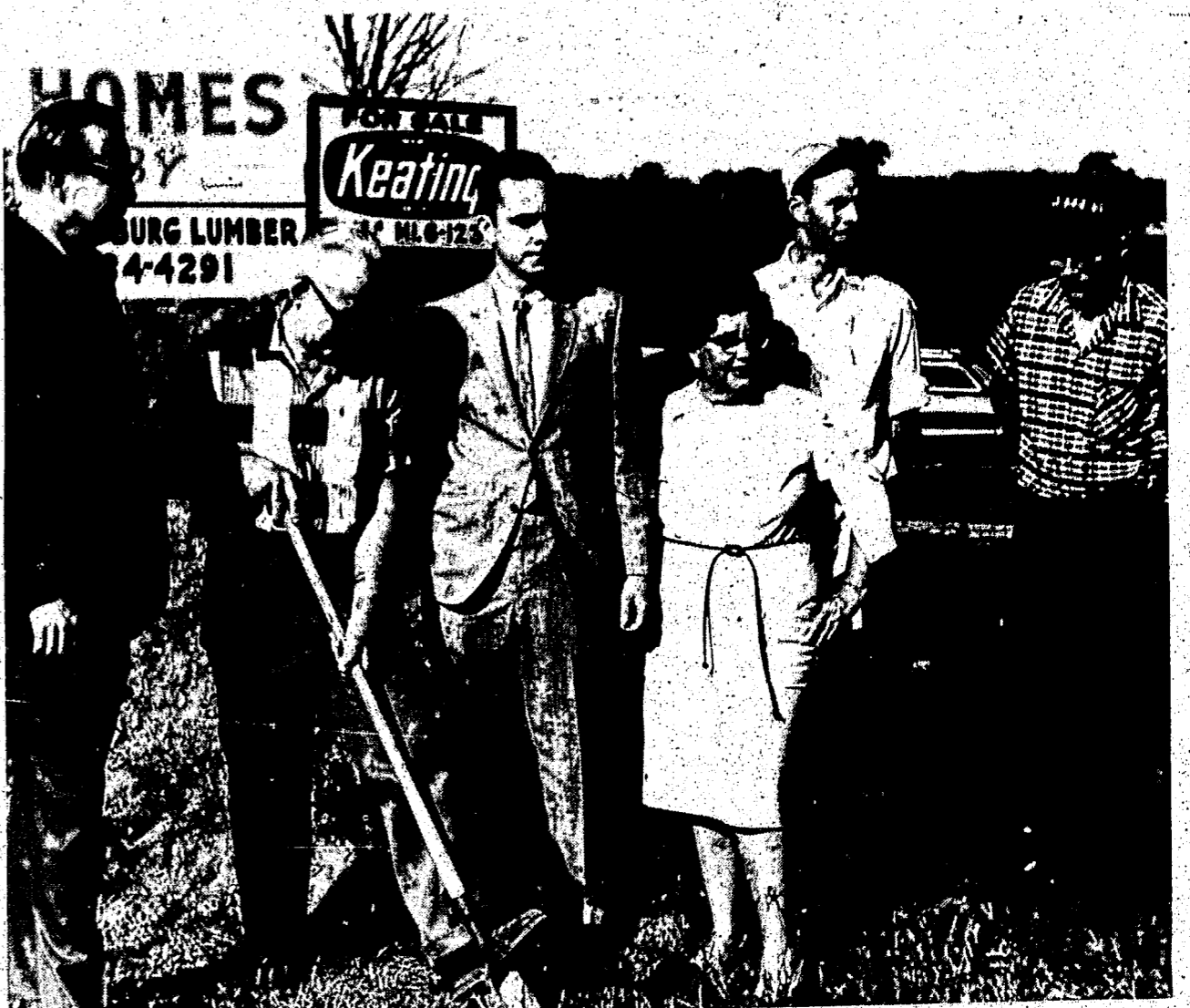
Shown at the ground breaking for a new house at Lake Braemar Estates are (from left) Arthur Jones, vice-president of H. T. Keating Co., developer; William Rogerson, owner of Lake Braemar; Robert Linebaugh, sales superintendent; Mrs. Clyde Nelséy, sales agent; and Marlin and Elwin Hillman, builders. Lake Braemar has more than 500 lots for home building. Of these, 120 are lake lots and the rest have lake privileges. The man-made lakes offer good swimming and fishing restricted to lot owners. An 18-hole golf course is also planned on the 400-acre property. Ten houses have already been completed and two more are under construction with completion planned in four months. Houses at Lake Braemar will range from $25,000 - $45,000.
