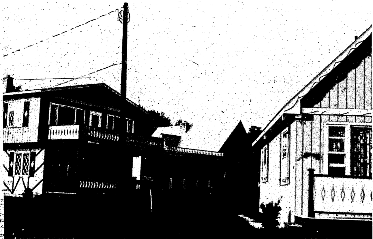
BUCKINEER—Left and right are chalets, 1 and 2 story, with the Buckineer Inn in the center. This $1 million area is on Portage Lake, Onekama.
