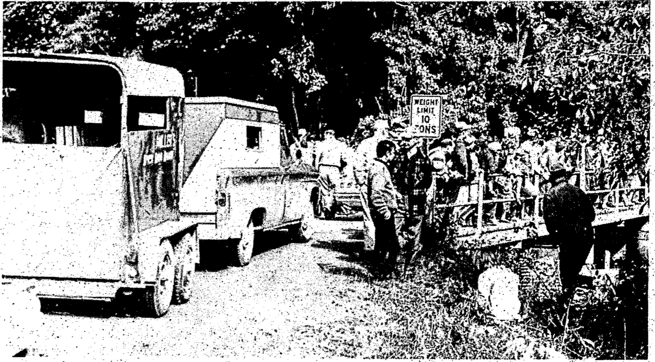
CROWDED BRIDGE — The 1-way bridge over Bear Creek truly was, especially with the number of people at the rails.
