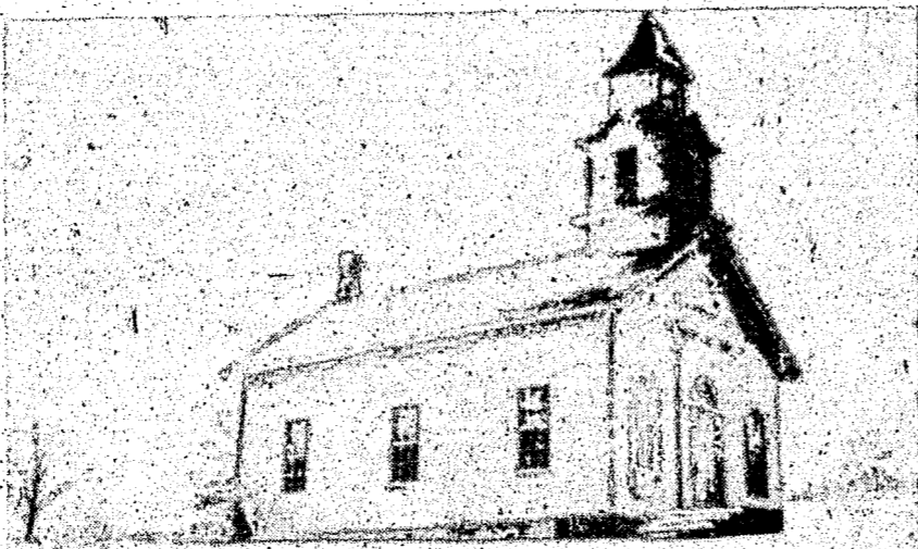
In 1870 the Mt. Bethel congregation replaced the original log church with a frame building.
