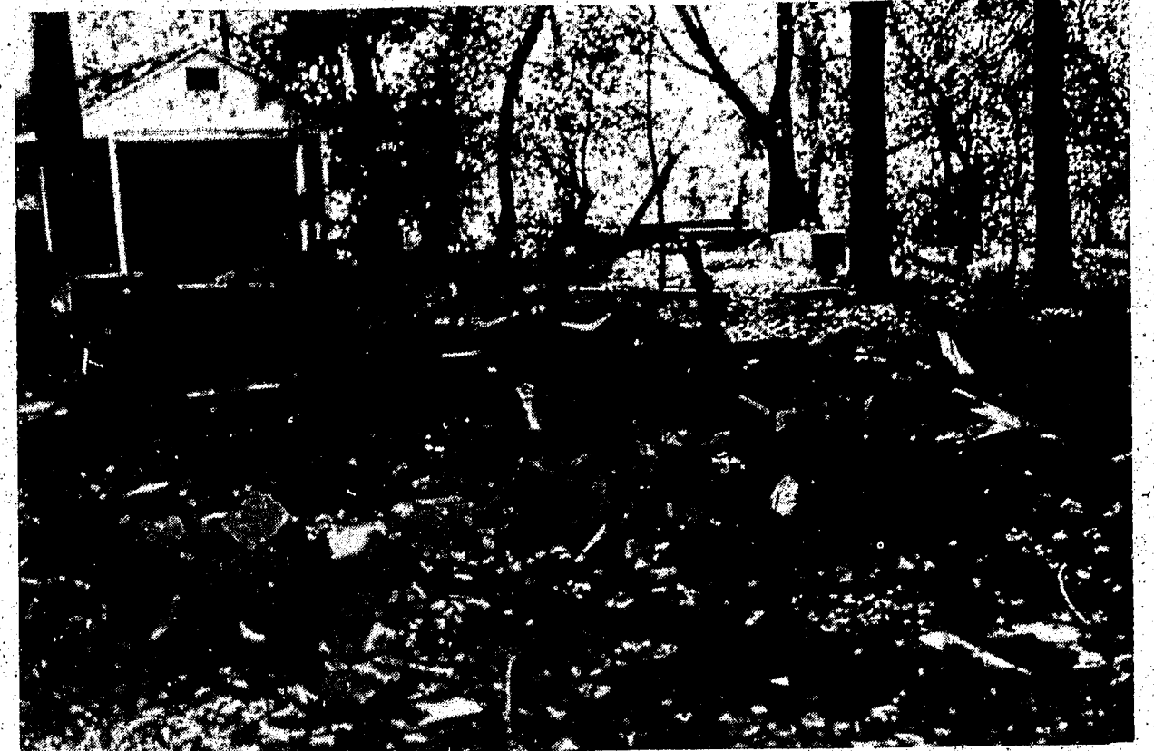
THE BURNED RUINS of what was once a garage still sits on its original site with no effort being made to remove it. It had been unused for several months when a car was pushed into it and set afire.
