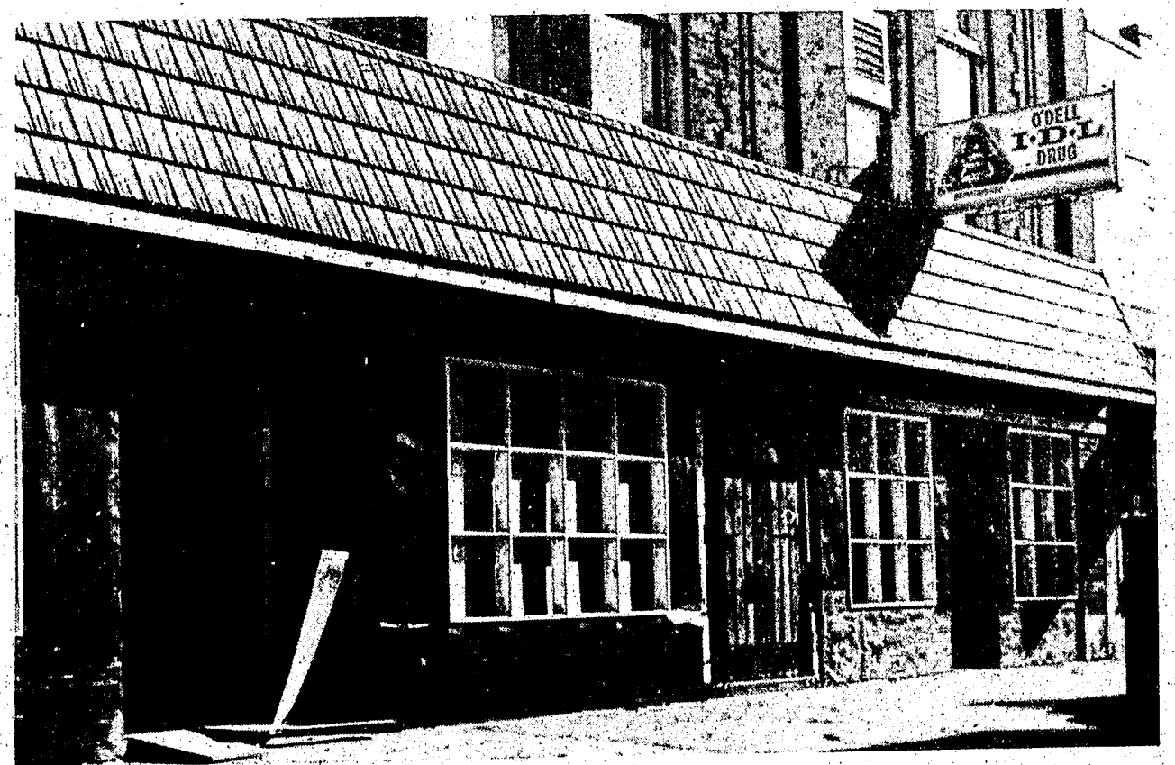
Clarkston residents and visitors have been amazed and thrilled with the fast rate of remodeling that is being done on the new section of town. Once occupied by the O'Dell Drug, Alger's Hardware and the Clarkston Bakery, present plans are for the expansion of the O'Dell Drug and the opening of a branch of the Richardson's Farm Dairy with a snack bar sideline.
