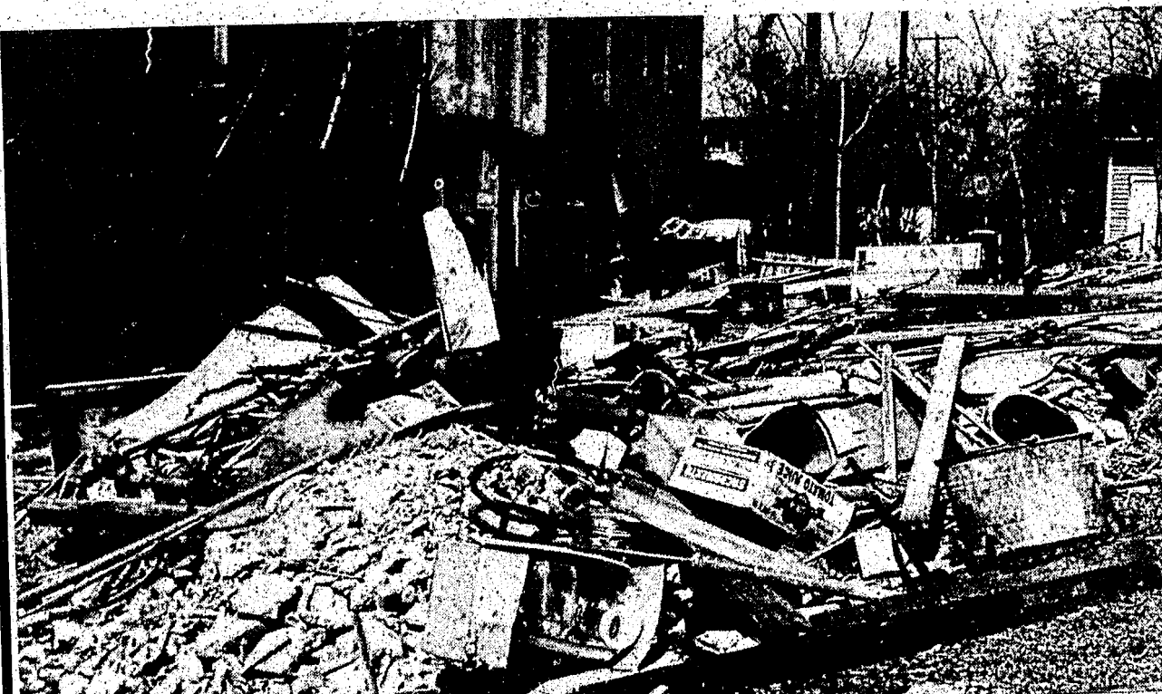
THE ALLEY looks a mess, and is, but it's temporary. The debris is what has been removed from what used to be the Clarkston Cafe building and O'Dell's Drug Store. Keith Hallman has now moved into his new drug store north of the previous location and workmen are remodeling the upstairs of the cafe building and waiting for plans for the downstairs where another restaurant is planned.
