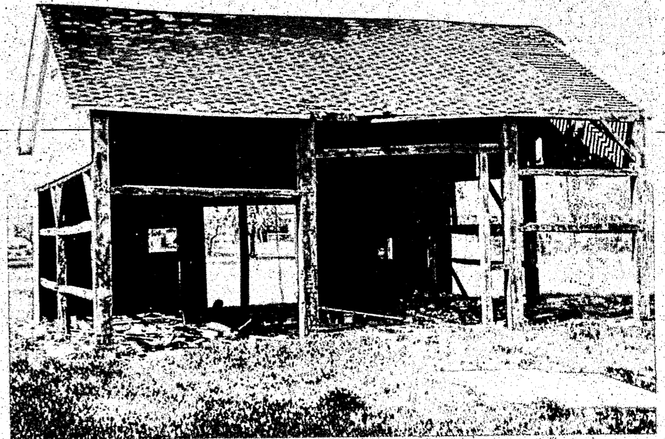
Standing stark and barren against the afternoon sun is this skeleton of a landmark that was once the property of an early Clarkston settler, Peter Addis. The barn is located on the property, now up for sale, of the Spenceley Butters' on Waldon road.
