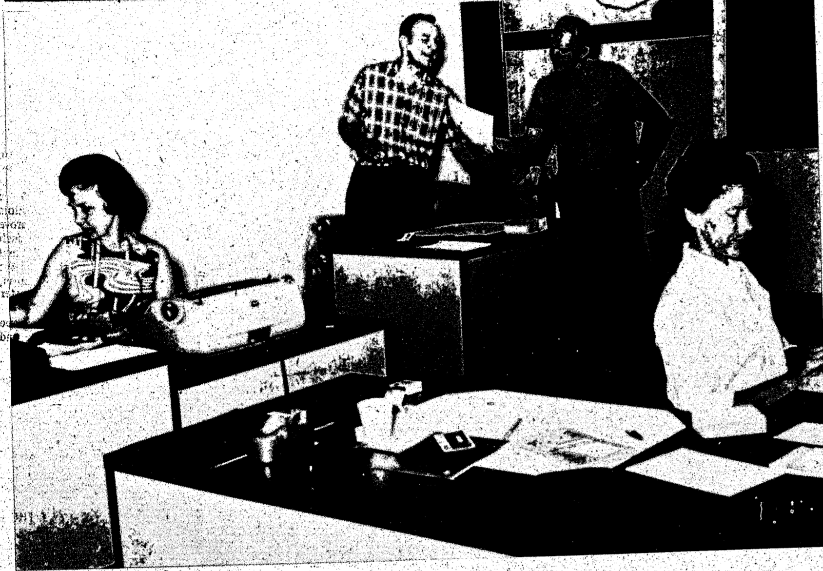
While construction work goes on, inside and out, at the new Junior High building, the monumental task of setting the front office in order begins. From left to right are Phyllis Mansfield, Gus Birtsas, assistant principal, Mel Vaara, principal, and Mary Ann Radoye, office secretary.
