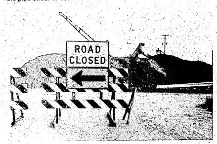
Problems arose when construction workers attempted to bore under Highway M-15 to install pipes. The pipes got bent by rocks and so it trailer. Earlier this year he sold was necessary to revoute the road and do some further excavating.
