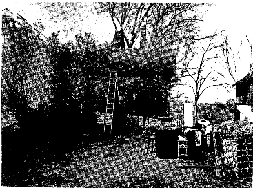
TOTAL LOSS — Last week Monday, just as the children were getting ready for school, fire broke out on the roof of this home at the corner of Clarkston and Baldwin roads. A family of 10 was left homeless. Some of the furniture was saved, but all the clothing was lost. Firemen from Orion are putting the last water on the ashes. Independence firemen assisted.
