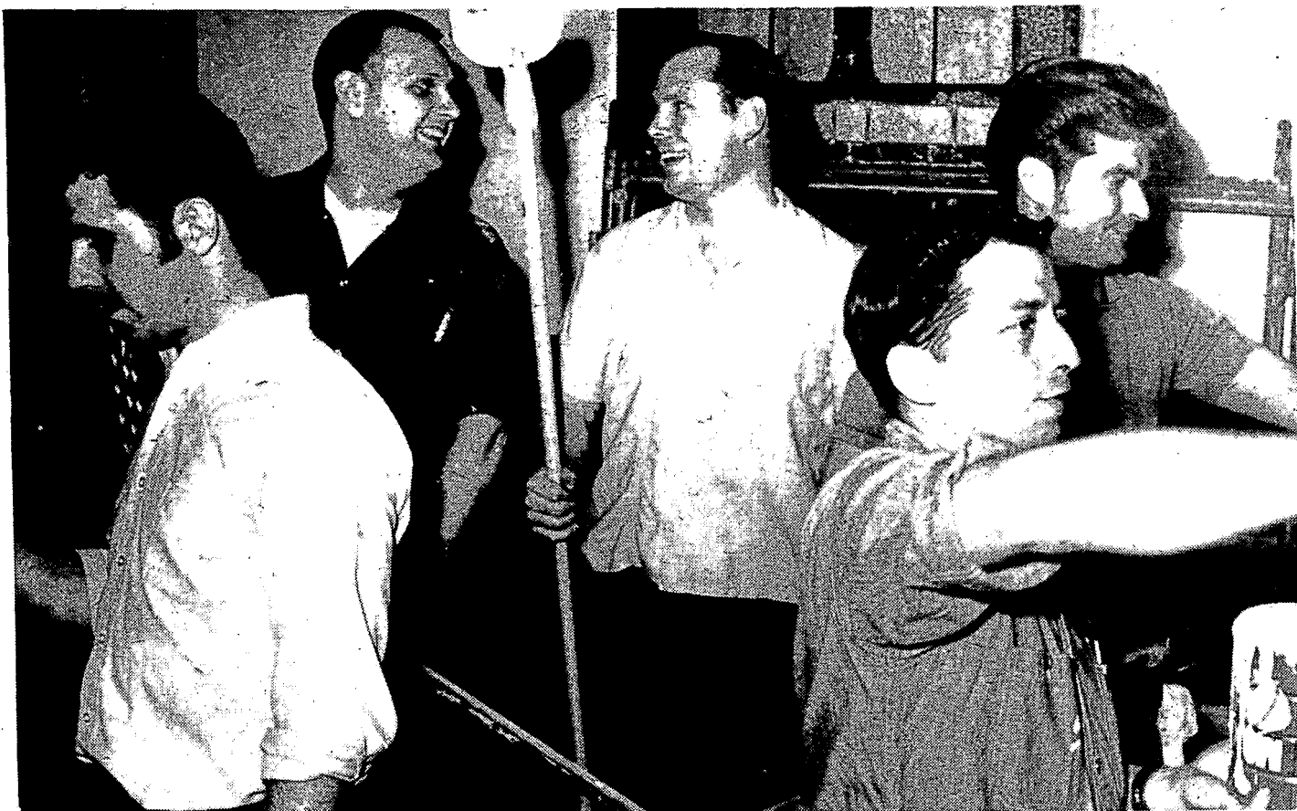
Jaycee first nighters used eleven gallons of paint, giving the Clarkston Salvation Army Citadel a spring lift. Working on the "inside job" and applying the paint, which was donated by John Garlac, are five second nighters. Left to right are Jaycee volunteer workers, Mike Madison, Jerry Bradley, Art Ripley, Harold Morgan and Larry Thompson.
