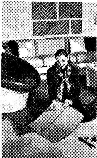
JUST PEEL AND place. That's all there is to custom shag floor coverings, when carpet tiles are used. These have self-adhering, latex foam backing.
