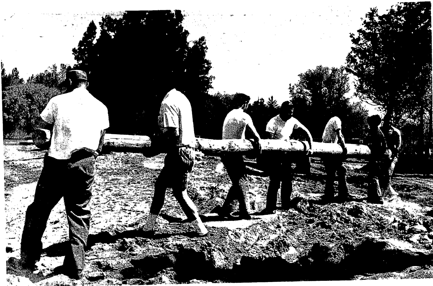
It takes a lot of manpower to handplace a big pole such as this which will separate sod and sand.
