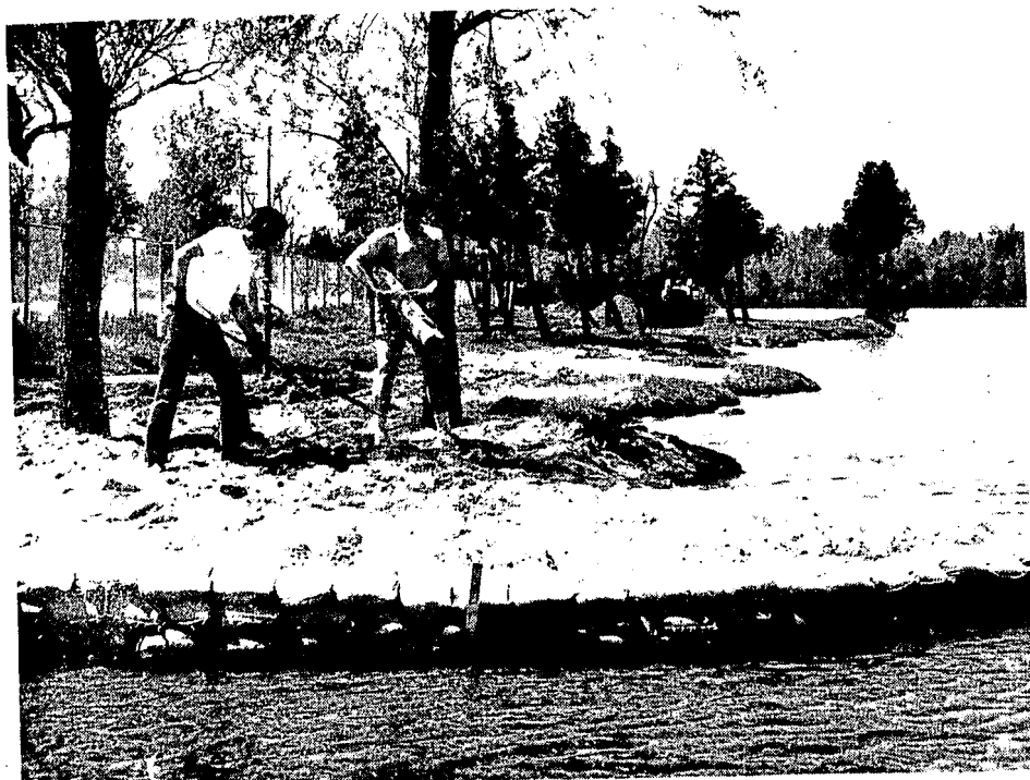
Ron Rule and Dave Nadolsky start work on the west end of the beach where erosion is still visible.
