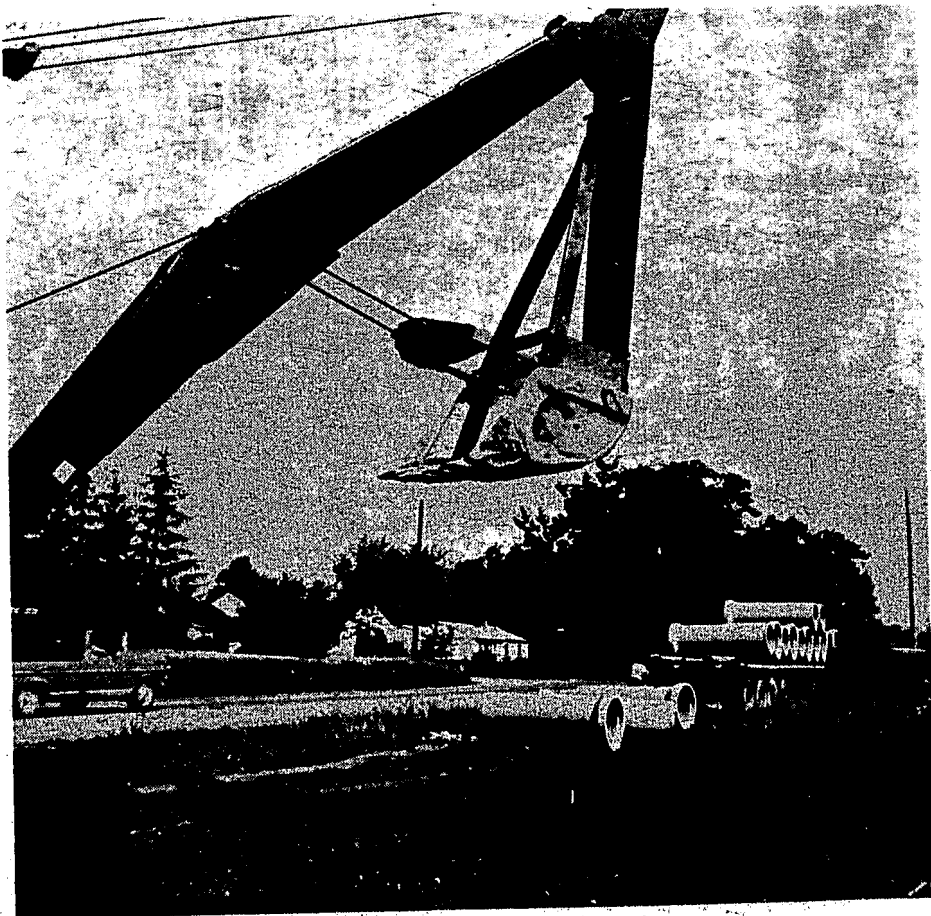
On M-15 giant trenchers divide the earth for positioning of sewer crock which will make-up the township sewer system. The trencher was at work near Princess Street.
