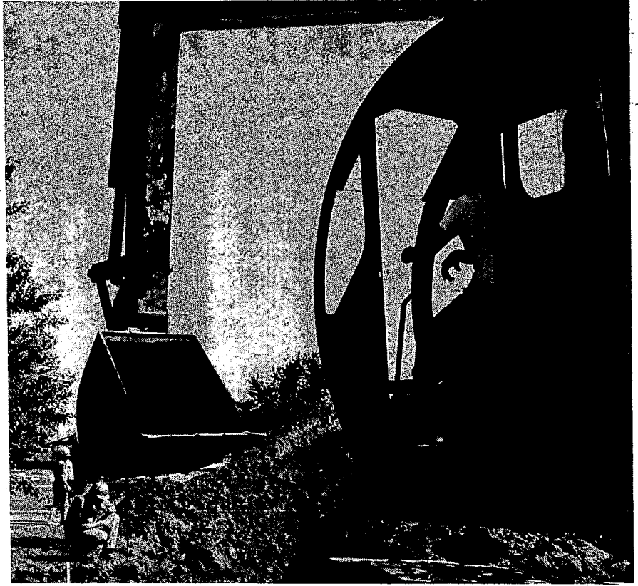
The sewers are coming.
