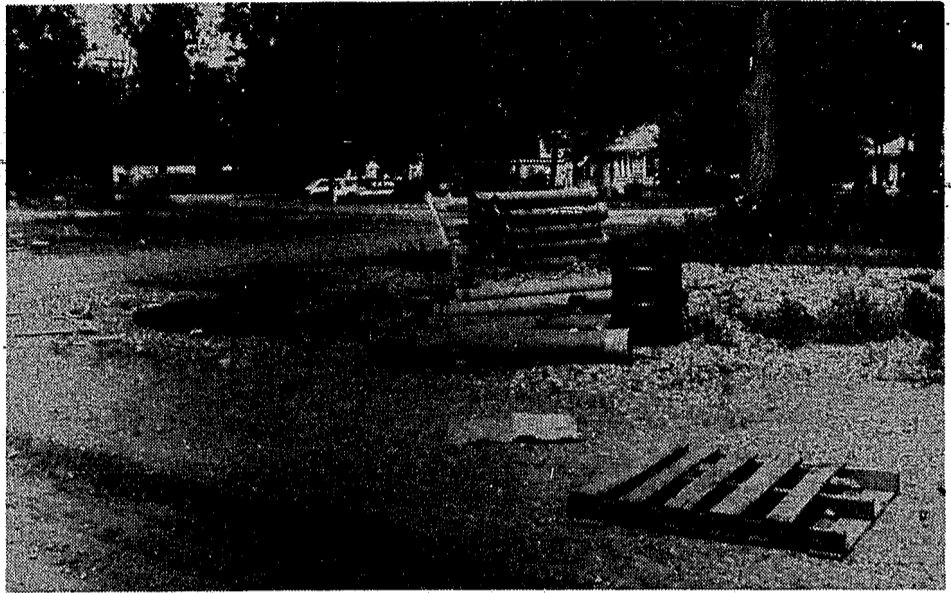
Litter left by sewer contractors on Park Street has made Woodhull residents unhappy.
