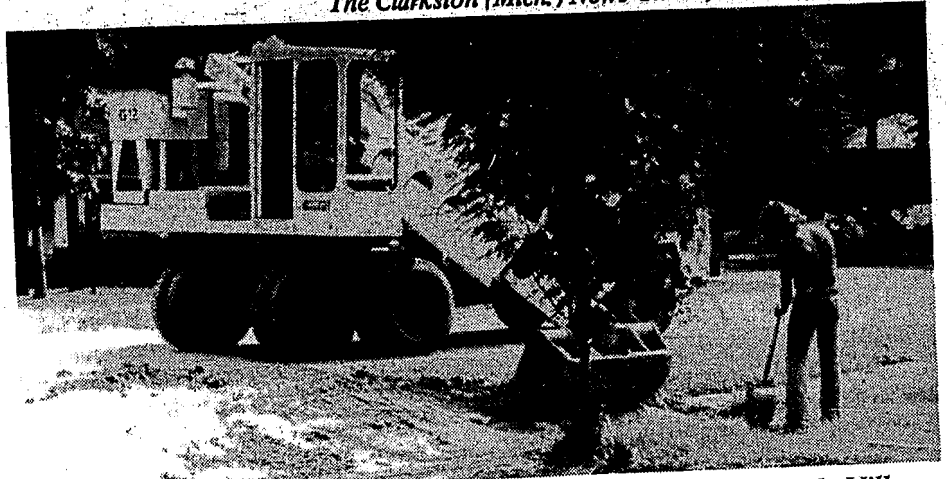
Contractors continue with their ditch-digging in Hi-Wood Village Subdivision, part of the restoration of property following sewer-line construction.
