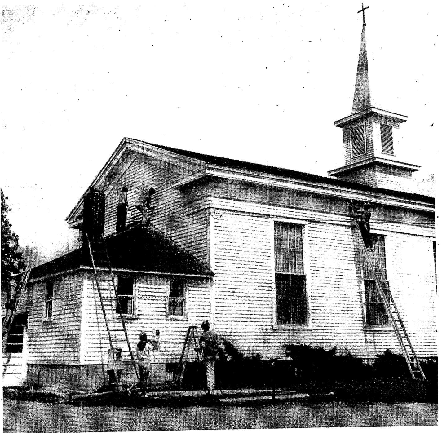
A drove of Clarkston Area Jaycees hummed around independence center Saturday, painting the exterior of the community building. Working against the threat of rain, they got the job about three-quarters done. They plan to finish it this Sunday. (See additional photos on Page 8.)
