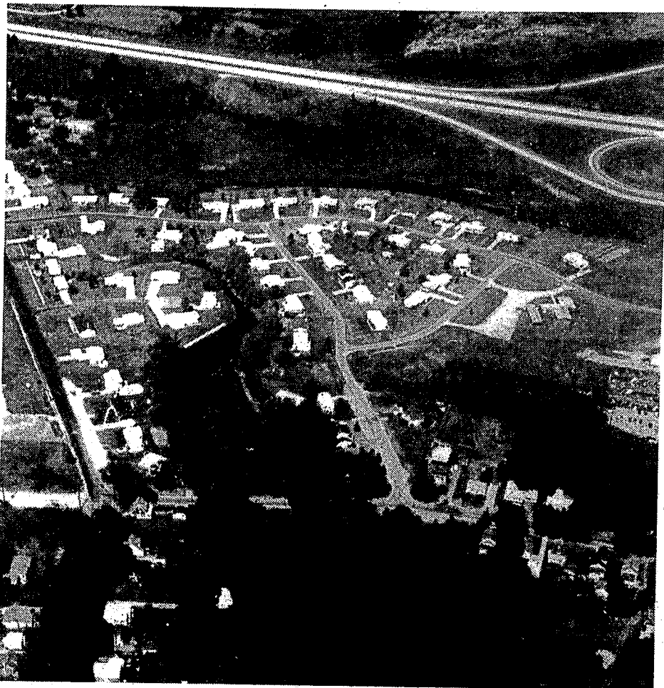
Pollution in the Upper Mill Pond shows clearly in this aerial view.
