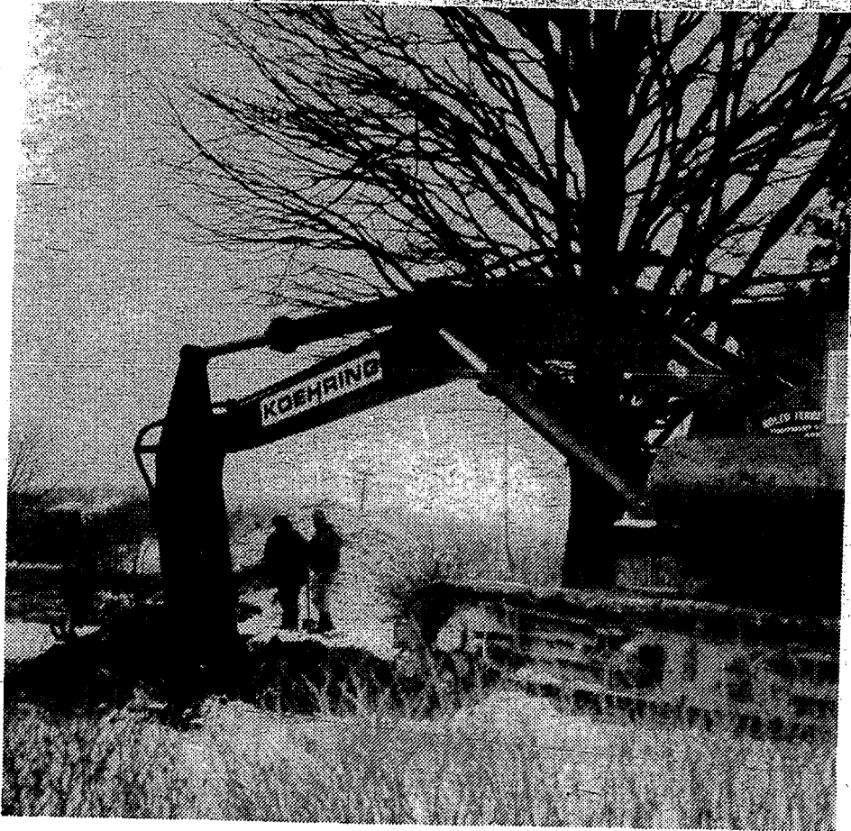
Workmen watch as giant machinery cut away the ground adjacent to the tree. A 20-foot pit was dug just three feet from the trunk.
