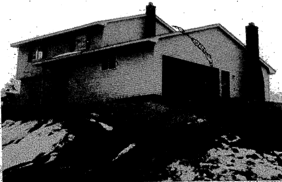
DeMasellis home nearing completion.
