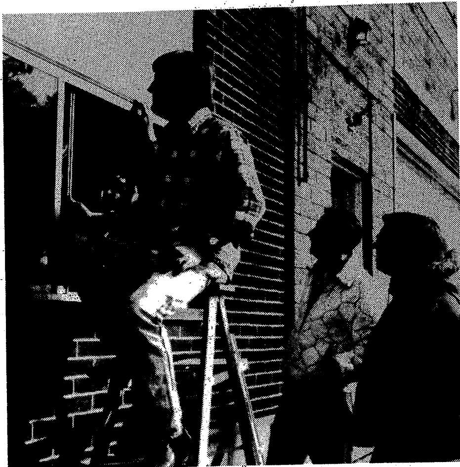
Kicking off a program to spruce up the Independence Township fire station in the village of Clarkston, volunteer firemen replace a cracked window.
