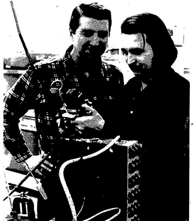
John Nicholson (left) of Clarkston and Charles Eastman of Waterford test a makeshift refrigeration unit put together in the major appliance repair course.
