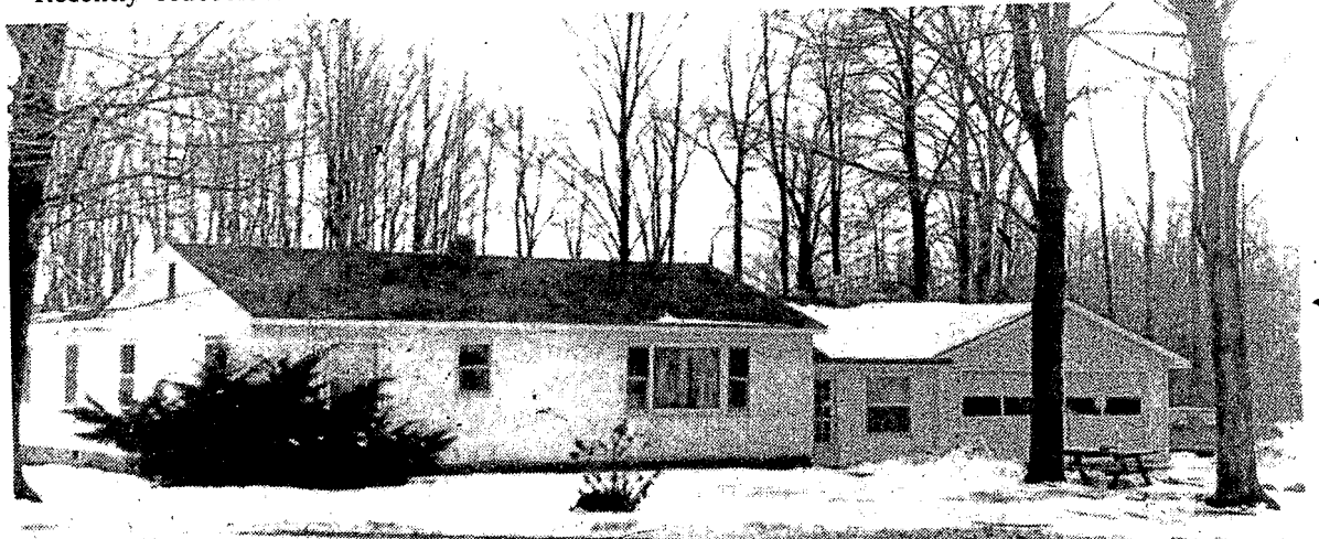
Trim house grew from inauspicious beginnings in the portion which is now the garage.
