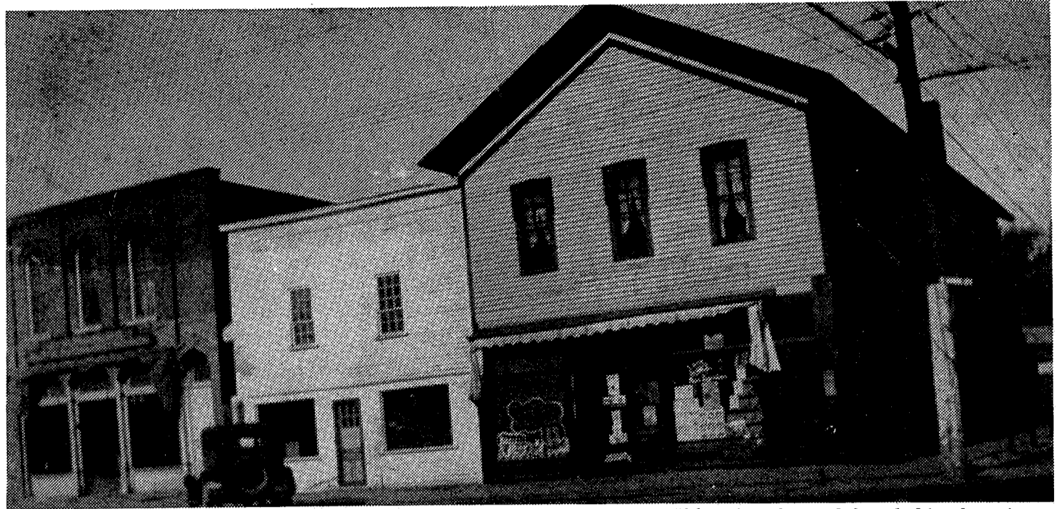
Gary Labenz of 7236 Holcomb Road found this photo in an old car he was reconditioning. It shows Rudy's Market when it was still located on the corner of Main and Washington and the barber shop belonging to Tug Barst. Both are gone now, burned in a fire in the 30's.
