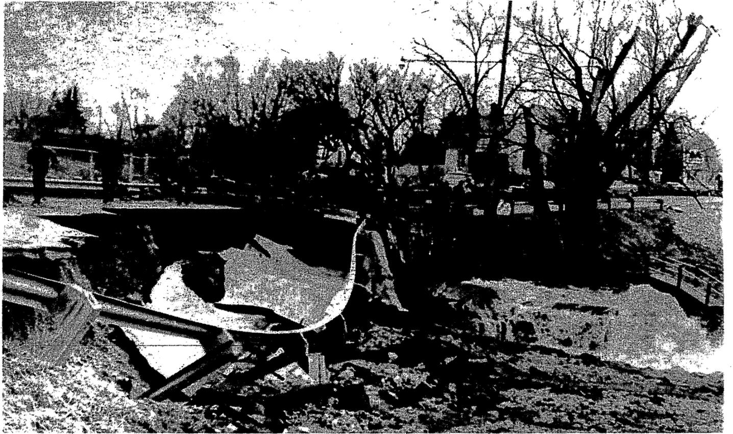
*Davisburg Mill Pond spillage eroded Davisburg Road, but sandbagging farther upstream prevented the dam from collapsing.*
