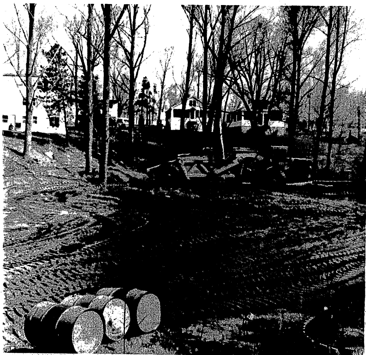
A 210 Michigan scraper levels the swamp off Lakeville in Walters Lake. The work is being accomplished in connection with the finish work on sewers by Armstrong Construction Co.
