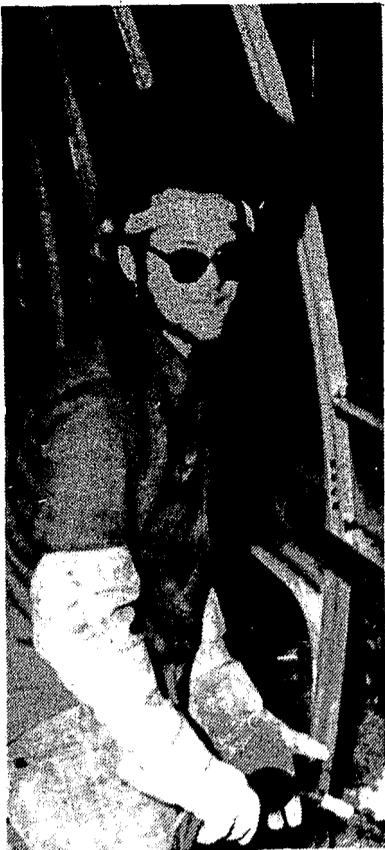
Dennis Novak of Sashabaw finishes welding a frame.
