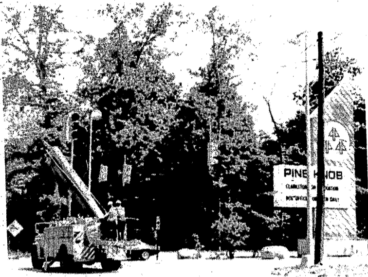
Workmen install traffic signals at Pine Knob entrance.
