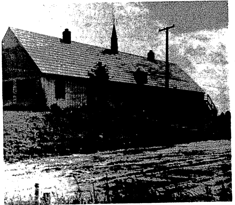
Tennis courts to be constructed here
