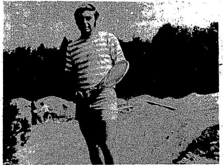
Work progresses on the addition at Deer Lake Racquet Club following ground breaking July 31. Completion date for the pool, exercise rooms, nursery, handball and tennis courts is set for October 1. "Since Forest is the builder it will probably be ready," said Henry Germain, tennis pro at the club, referring to Forest Milzow, owner of the club. The restaurant will be finished at a later date.
