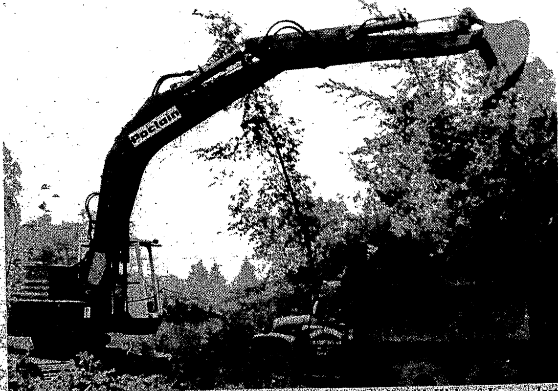
The construction firm of Clement and Kirk of Lapeer last week began work on Clarkston's new Post Office, to be erected next to the Dairy Queen on M-15. Workmen here excavate along the highway.
