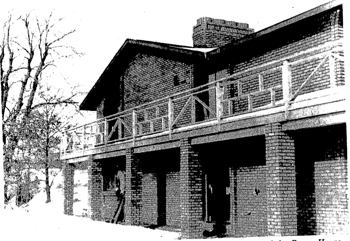
Exterior of the Rouse House.
