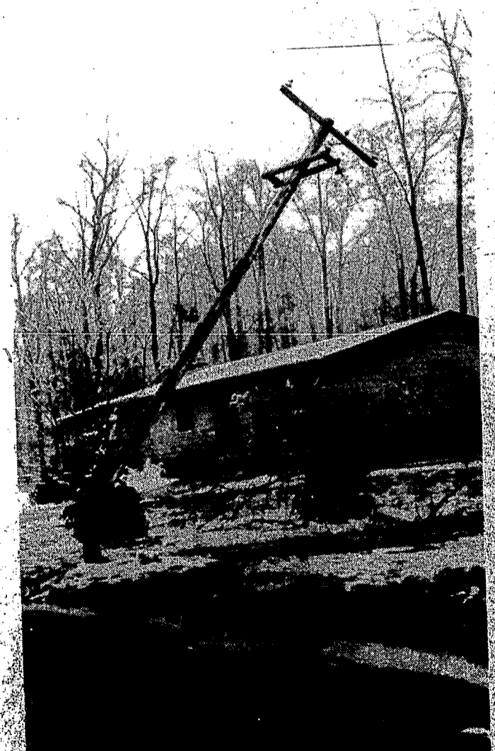
A telephone pole sheared by the weight of the lines in front of the Lowell Satterlee home, 5996 Hummingbird.
