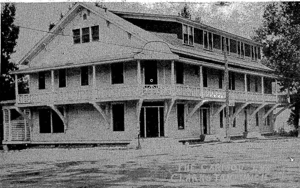
Caribou Inn after remodeling. The third floor is finished, with dormers and braces replacing the post on the ground floor porch. Photo courtesy of Mrs. Jack Haupt.
