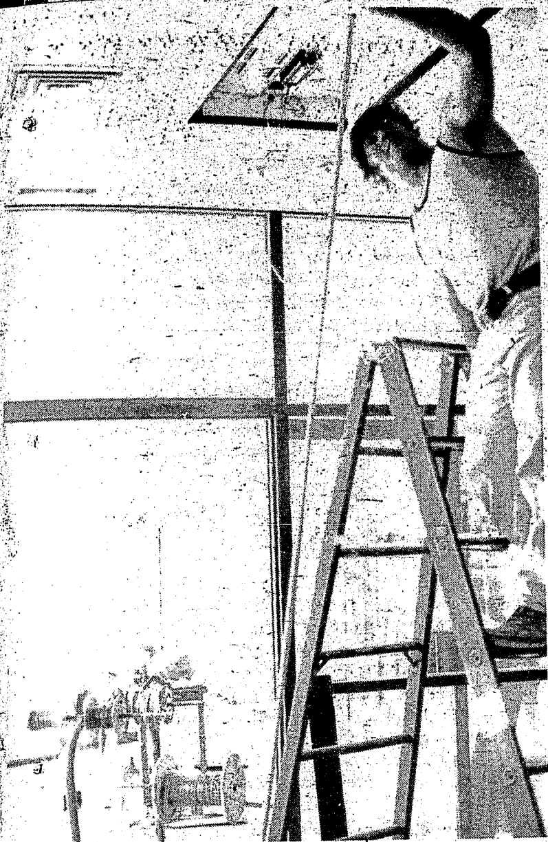
Postmaster Ray Klein hopes to move his Clarkston office into these new quarters on M-15 south of the village by next Monday. Contractors are now finishing interior work on the building. The old Post Office in downtown Clarkston will become lawyer's offices after the switch is made.
