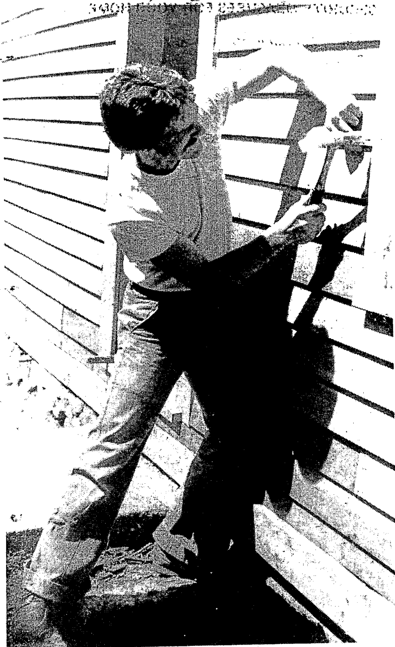
Bob Adams repairs siding on old green house on Buffalo Street.
