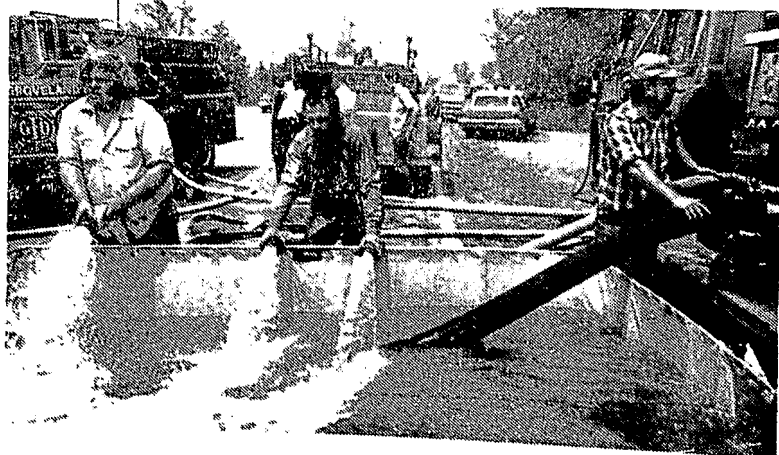
Volunteers man a water transfer tank.
