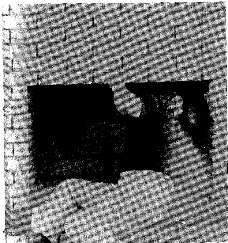
A normal day has Curn looking up a chimney checking the flue...
