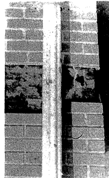
This particular patch of brick was replaced only last week.
