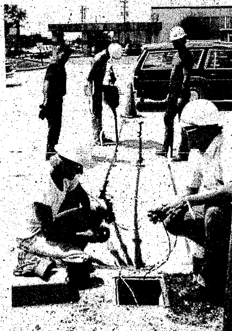
INSTALLING TRAFFIC ACTUATED TRAFFIC SIGNAL. John Leonard, left-front; Stephen Maku-shik, right-front; and Kenneth Bredow, Bob Reiten and George Michaels of the Road Commission's traffic department bury sensor cables under Southfield Road. The cables will help regulate a signal at the intersection with 10 Mile Road, enabling through motorists more time when there is no left-turn traffic, and enabling safe left turns when there is a demand.
