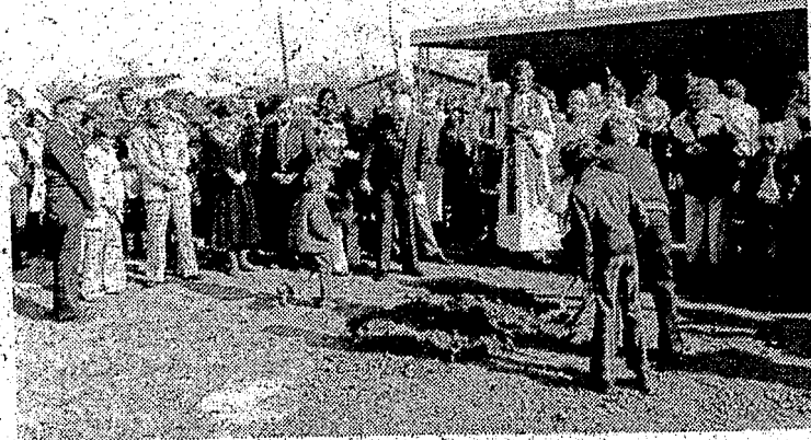
Pastor Robert Walters and the congregation of Calvary Lutheran Church turned out in force last Sunday as the ground breaking ceremony for the new church addition got under way.
