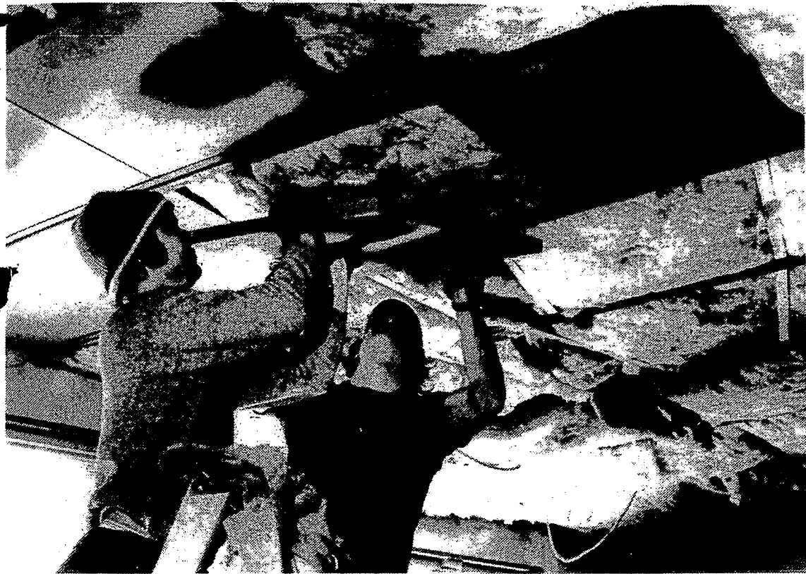
The flanges of bar joists are used to support Sol-Ar-Tiles. Each tile weighs 43 pounds and can release approximately 465 BTUs of heat over a 10-degree cooling range.
