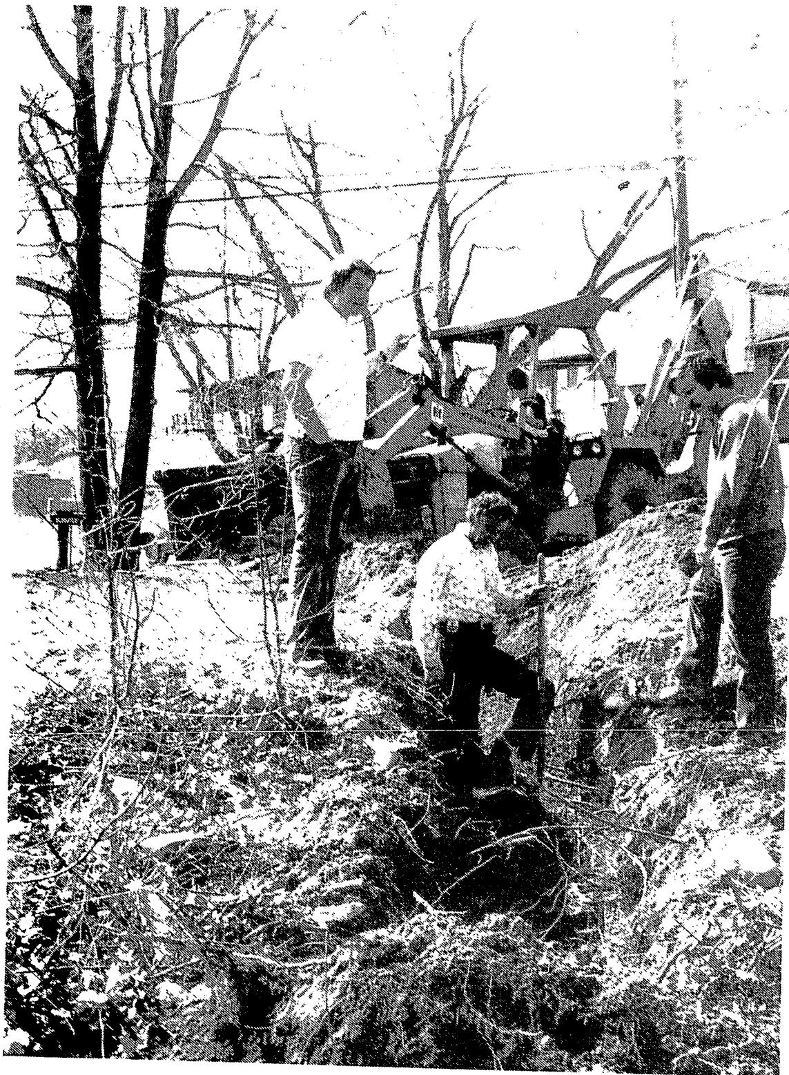
A culvert under Algonquin, part of the current road improvement work being done in Thendara Park, gets the once-over from one of the subdivision's former road chairmen, Bruce Walker [left], and the man who now holds the job, Len Nowak [right]. Subdivision property owners are paying to have two culverts put under the road and to have a sharp curve straightened.
