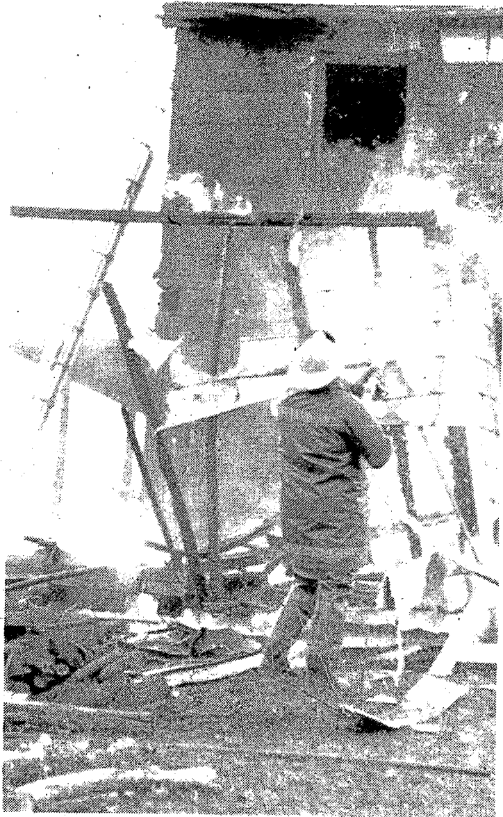
Fire at Sheehy home spread to second story.
