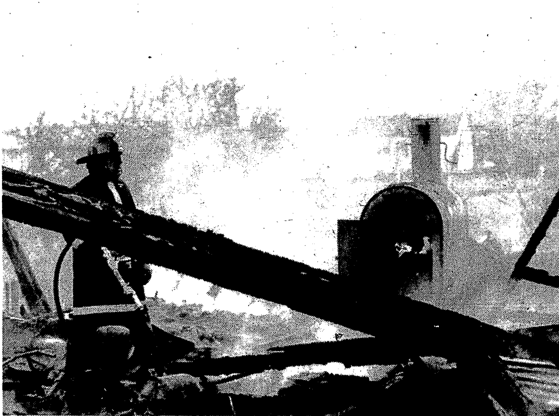
Amid smouldering ruins of garage, fire in incinerator crackles on. Photos by Pat Braunagel
