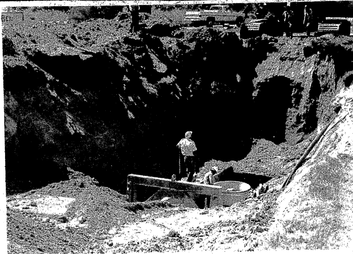
Construction workers finish the main outlet for the Deer Lake Farms sewer system. The 15-foot deep hole was completely covered the next day.
