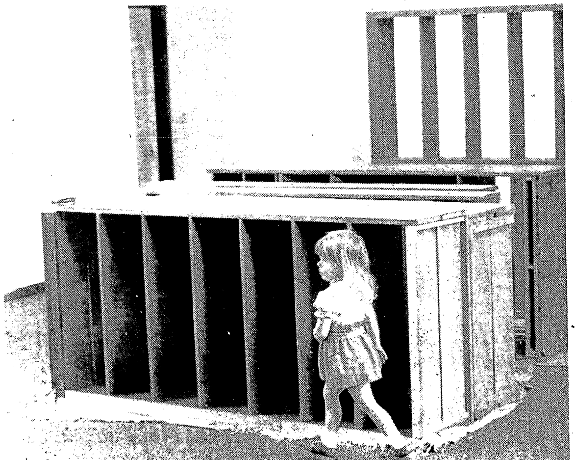
Strolling by bookless bookshelves lying on their sides, 3-year-old Kathy Jackman tours the new Springfield Township Library while her father Tom does some of the electrical work needed to be completed before the library can be opened.
