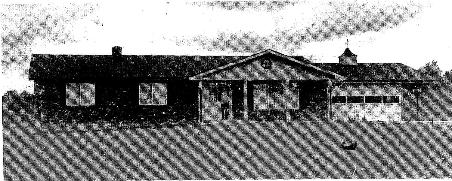
Located in the Shiawassee Creek Farms subdivision in Springfield Township, this house will be the home of six handicapped residents, at least until the court rules on a
